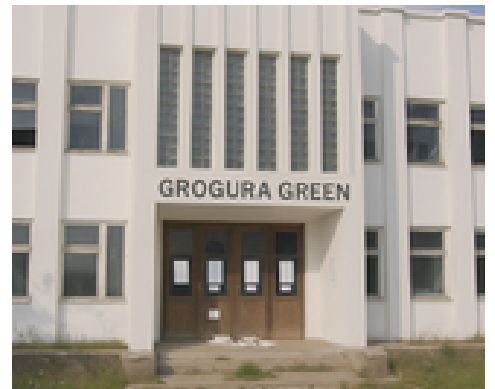
The abandoned Grogura Green Office complex with notices posted on the door--Photo: The Mustafar Enquirer
